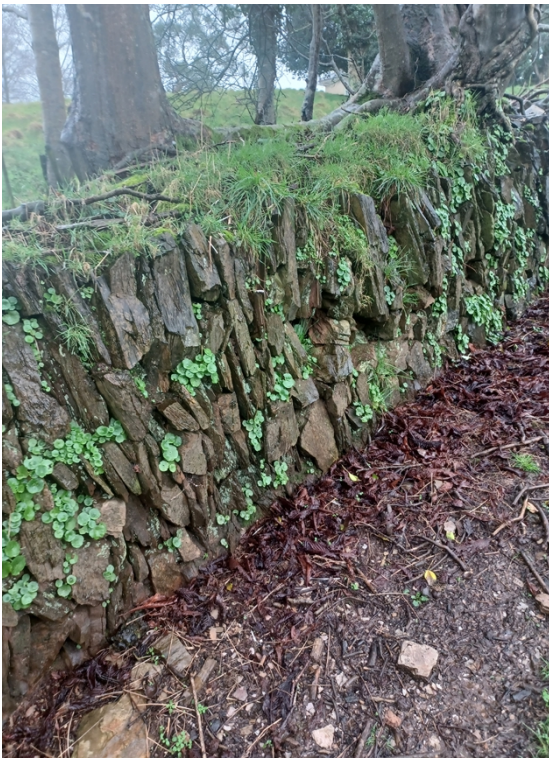
Towards point B and temporary diversion
