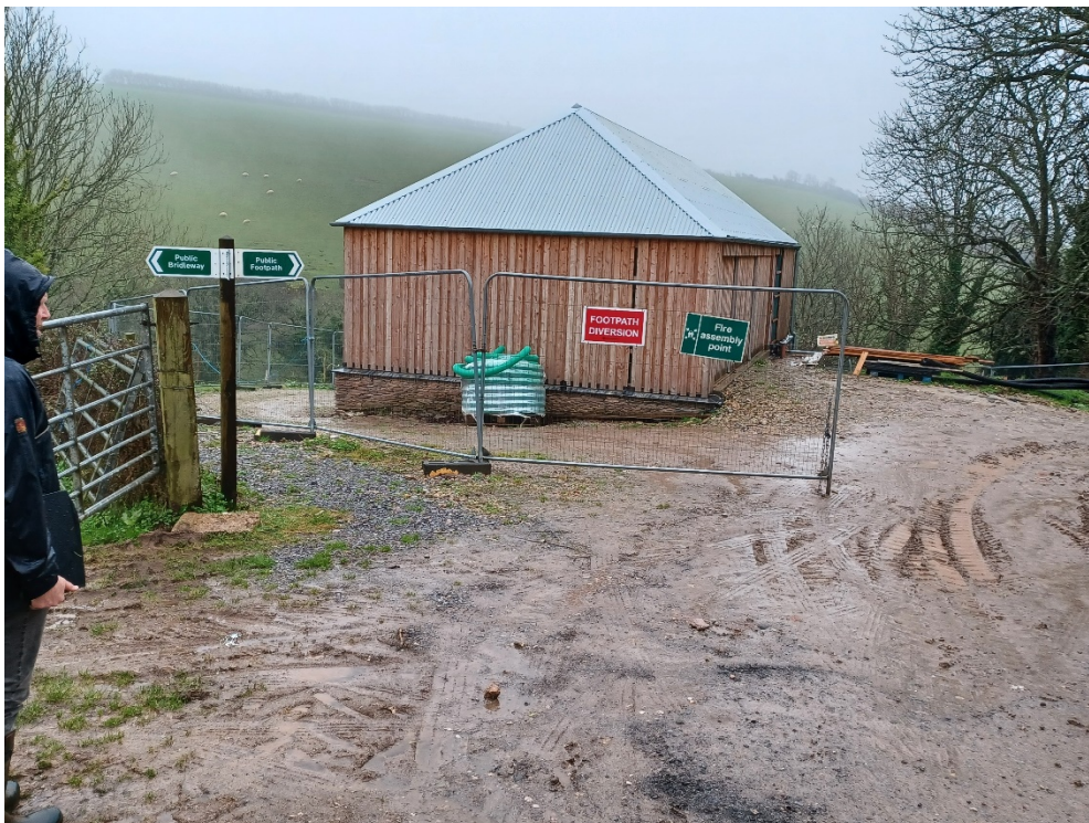
Finger post at point C junction with Bridleway No.12 Thurlestone and new barn
